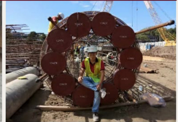
Bored Pile BP2400Ø
