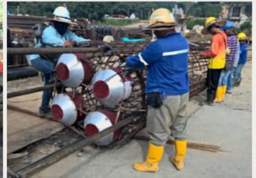
Bored Pile BP1500Ø
