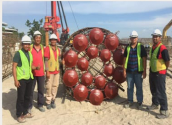
Bored Pile BP2200Ø
